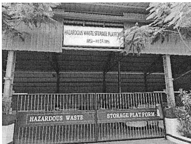
Hazardous Waste Storage Unit
