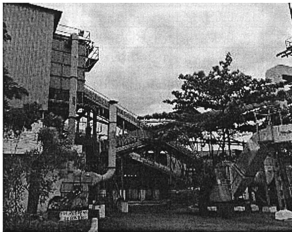
Coal Handling area – Conveyor belts with closed shed
